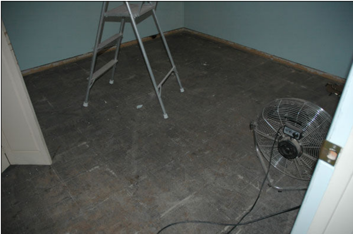
Heavy Mastic on the floor under the tile in the extra bedroom
