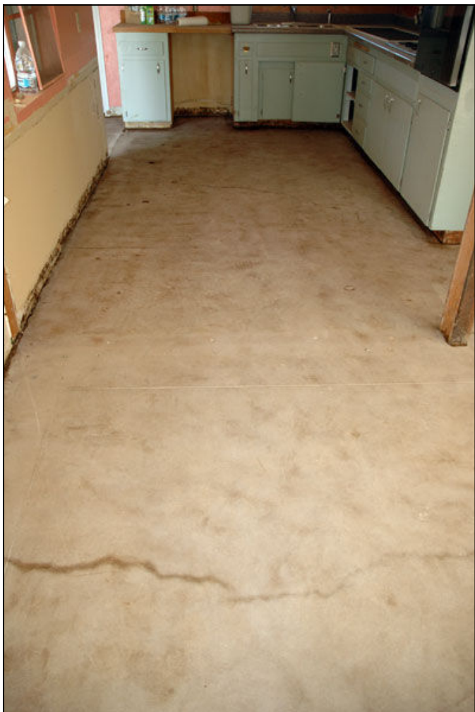
Kitchen After the Removal
