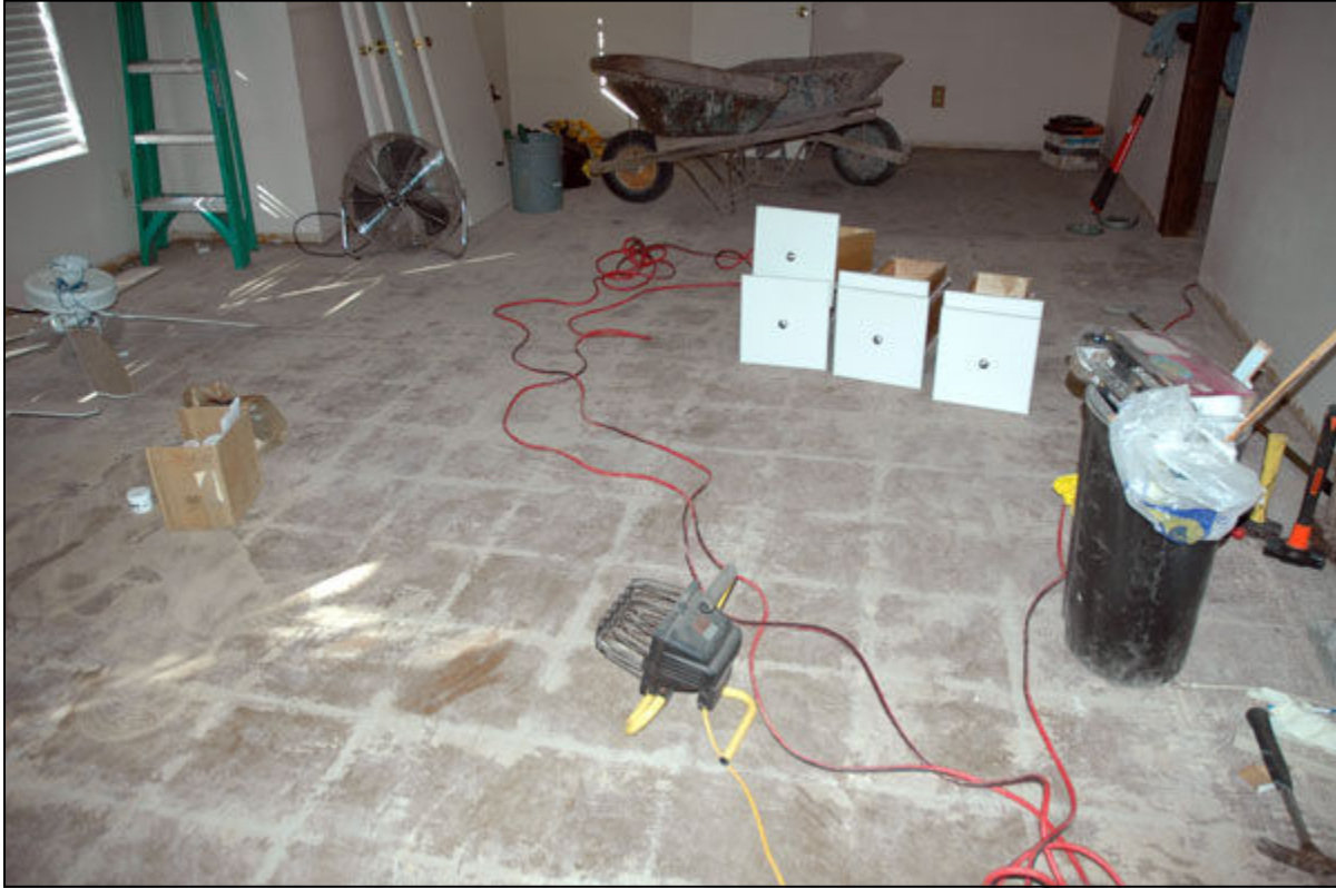
Heavy Mastic on the floor under the tile in the extra bedroom
